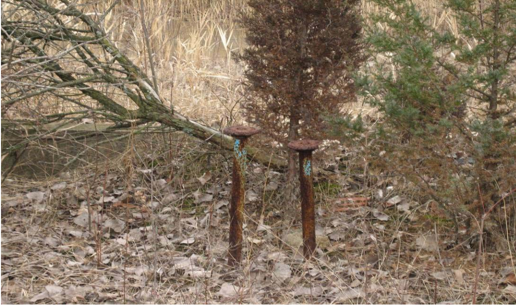
View of Installed Water Main Shut-offs
